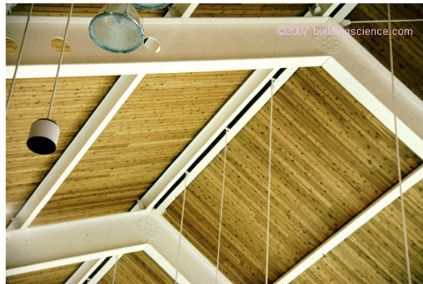
Photograph 4: Compact Roof For Pool Enclosure
