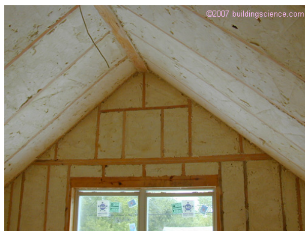
Photograph 2: Spray Foam Insulation
