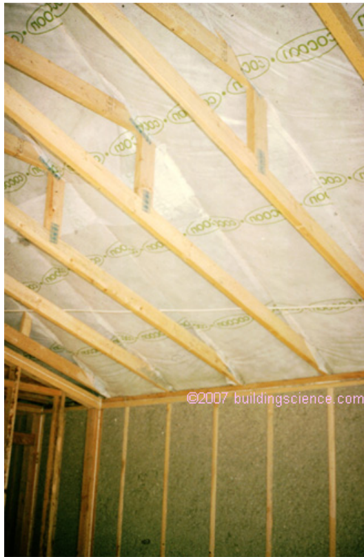
Photograph 3: Netted Cellulose – air and vapour permeable insulation in hot-dry climate.
