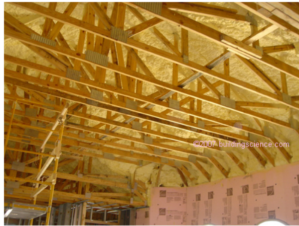
Photograph 5: Typical low density spray foam
